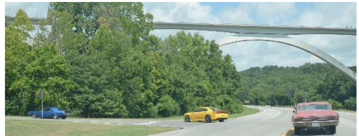
Natchez Trace Parkway bridge outside of Franklin, Tn.
